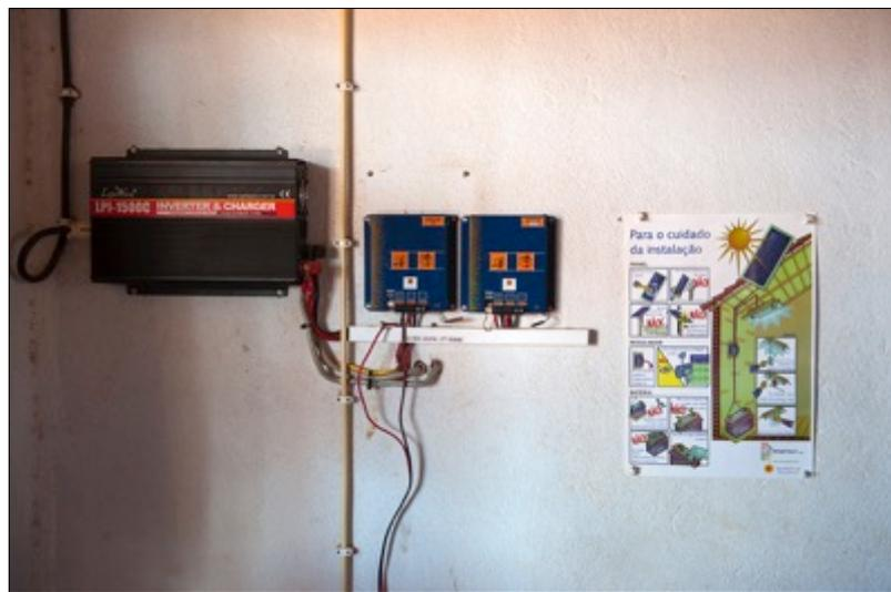
**Photo 9: Image of a solar power system for refrigeration in the Clinic, Massingir Velho**
